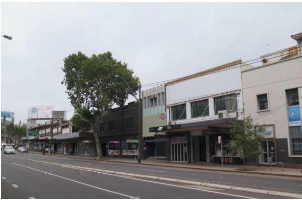
Figure 18 – Subject site with view of two-storey, commercial buildings located on the eastern side of the Pacific Highway – from right to left, Nos 395-397, 399, 401-5 and 407 Pacific Highway.
