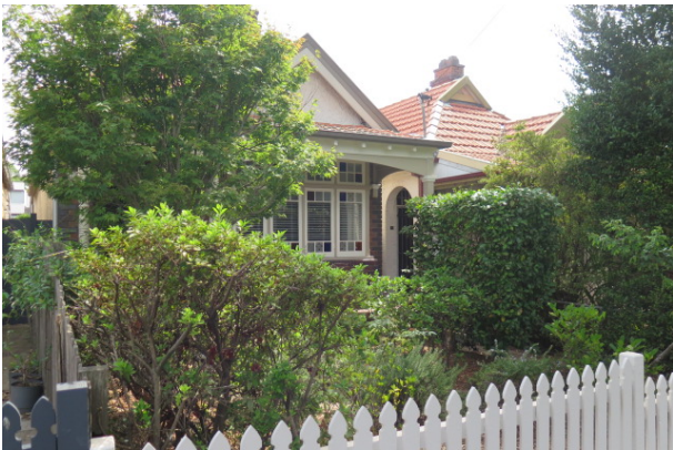
Figure 40 – Single-storey dwellings in Burlington Street, within the Holtermann Estate B HCA
