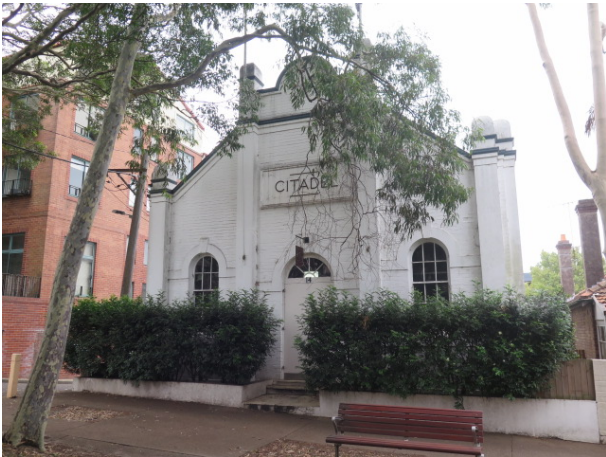
Figure 30 – Former Hall, located at 14 Hayberry Street, Crows Nest, is a heritage item located east of the subject site within the Holtermann Estate C HCA.
