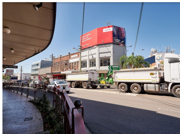
Figure 75 – View towards the subject site from the main entry of the heritage item, Crows Nest Hotel, showing there will be direct views to the proposed development
