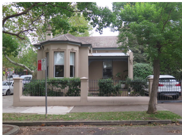
Figure 39 – House at 18 David Street, is a heritage item within the Holtermann Estate C HCA .
