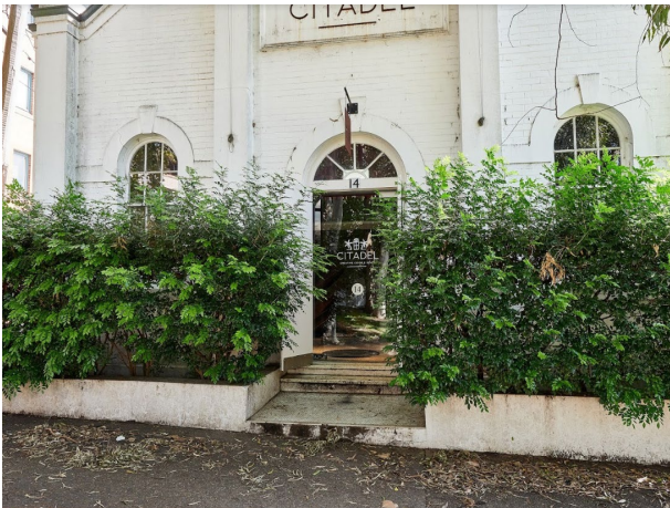
Figure 86 – View of entry to heritage item at 14 Hayberry Street, located within the Holtermann Estate C conservation area
