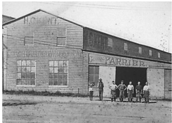
Figure 52 – HG Kent coachbuilding & wheelwright shop, Crows Nest, c1908 Source: North Sydney Heritage Centre Collections Station Library, LH REF PF832
