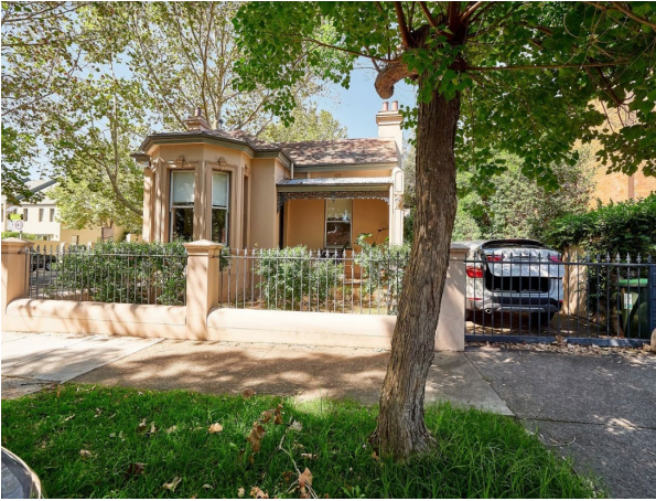
Figure 88 – View of main entry to heritage item at 18 David Street within the Holtermann Estate C conservation area
