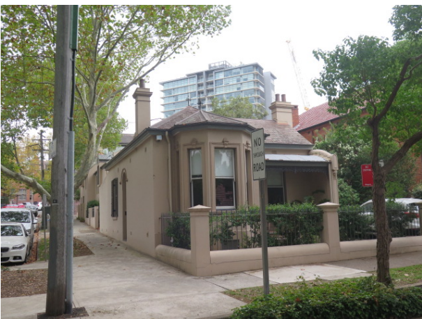
Figure 38 – House at 18 David Street, is a heritage item within the Holtermann Estate C HCA showing an existing high-rise development located in the background. It is possible the proposed development will be visible in the distance to the northwest of the principal entry.
