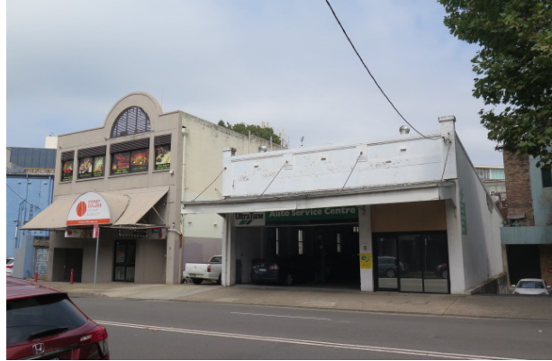
Figure 27 – No 6 Alexander Street (left) is a two-storey, late-20th century commercial building. No 8 Alexander Street (right) is single-storey motor mechanic shop, possibly dating to mid-20th century.
