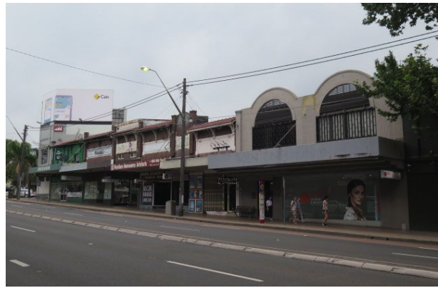
Figure 19 – Subject site with view of two-storey, commercial buildings located on the eastern side of the Pacific Highway – Nos 407, 409-419 and 423.
