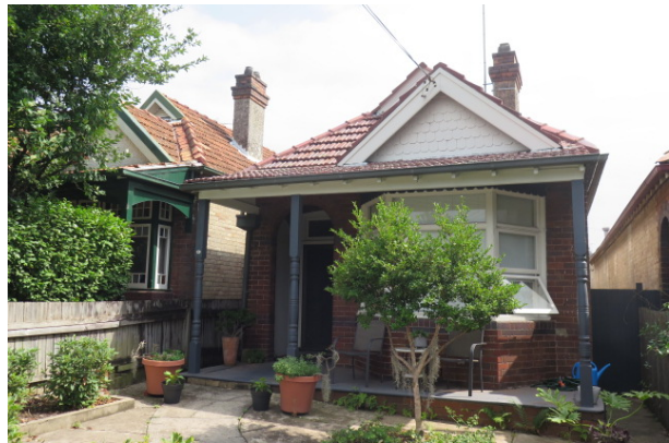
Figure 41 – Single-storey dwellings in Burlington Street, within the Holtermann Estate B HCA
