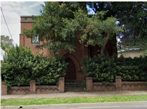
Figure 82 – View of main entry to heritage item at 69 Falcon Street located east of the subject site
